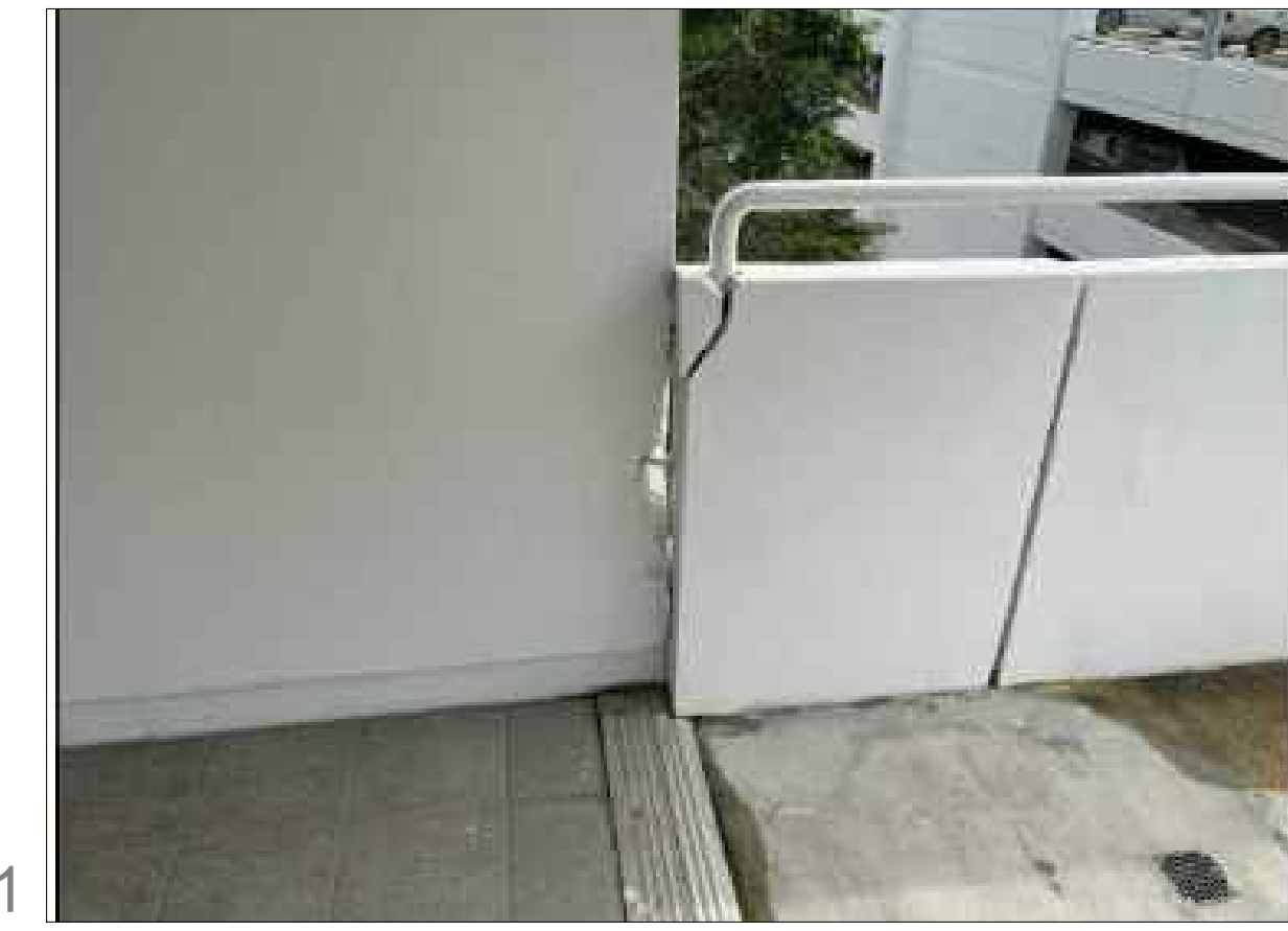
SIXTH FLOOR GENERAL VIEW
