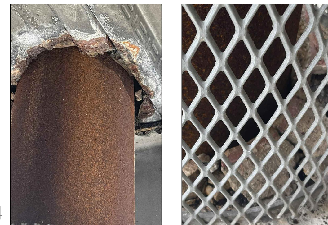
DAMAGE 3 BEAM CORROSION, IN THE BRIDGE AREA BETWEEN BUILDINGS. THE REPLACEMENT OF THESE IS RECOMMENDED.
