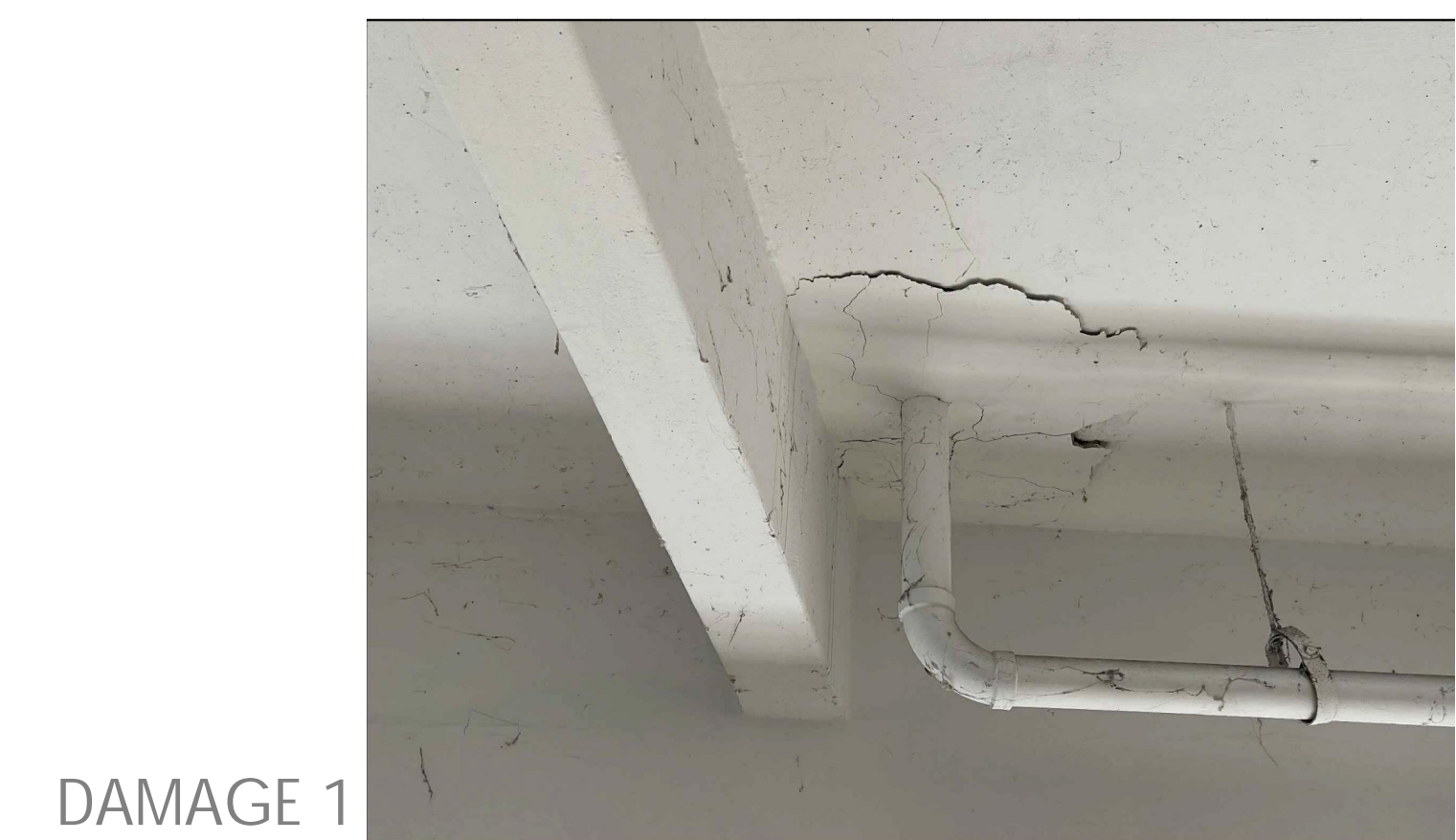
CORROSION OF CONCRETE SLAB AT CORNER
