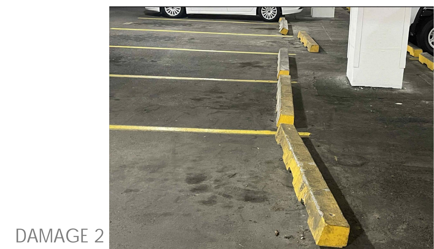
WHEEL-STOPS WITH INADEQUATE SUPPORT
