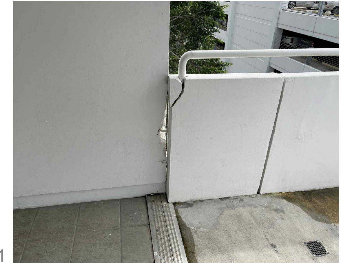
SIXTH FLOOR GENERAL VIEW
