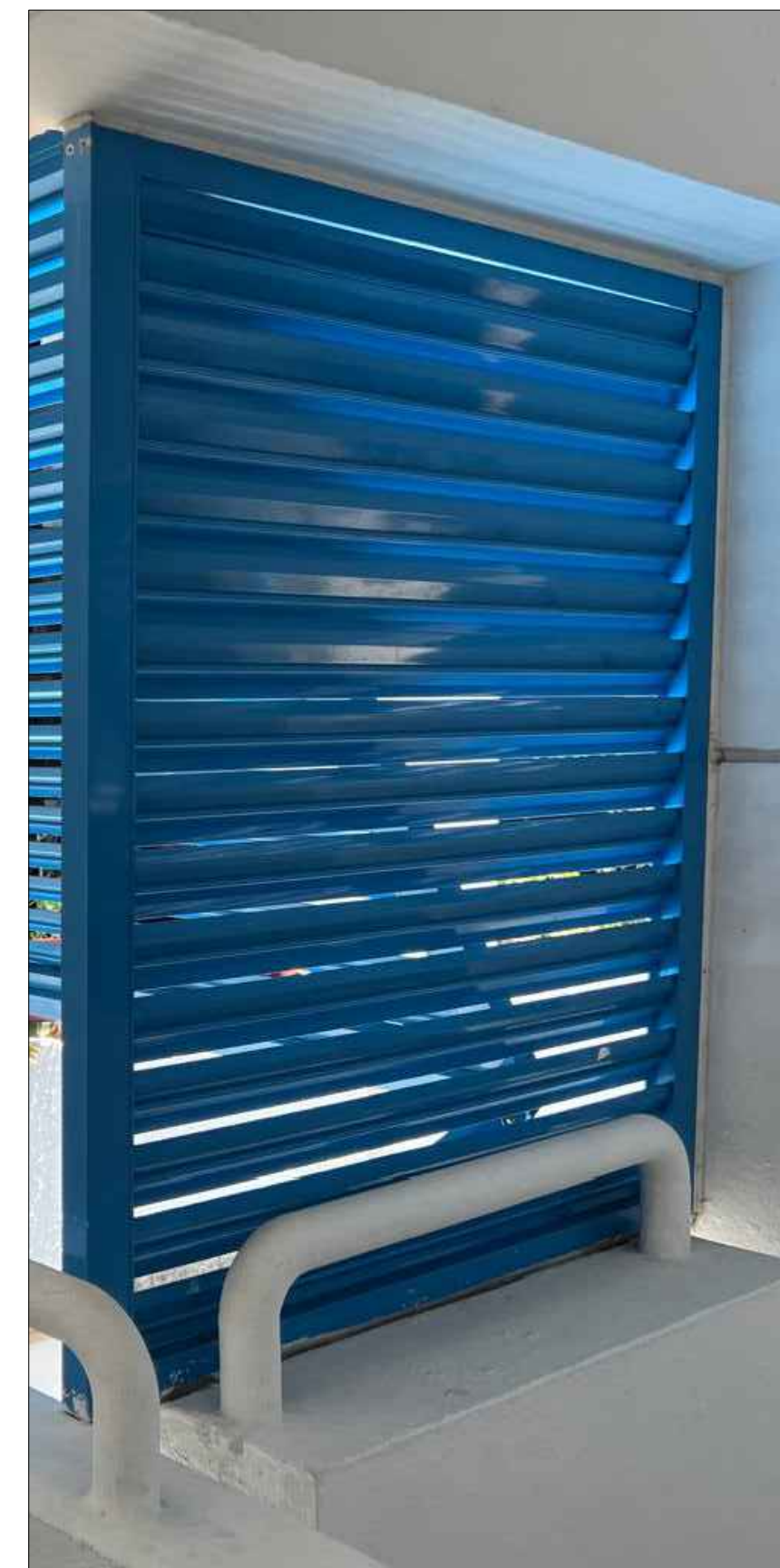
DETAIL 2: METAL FIXED LOUVRES
