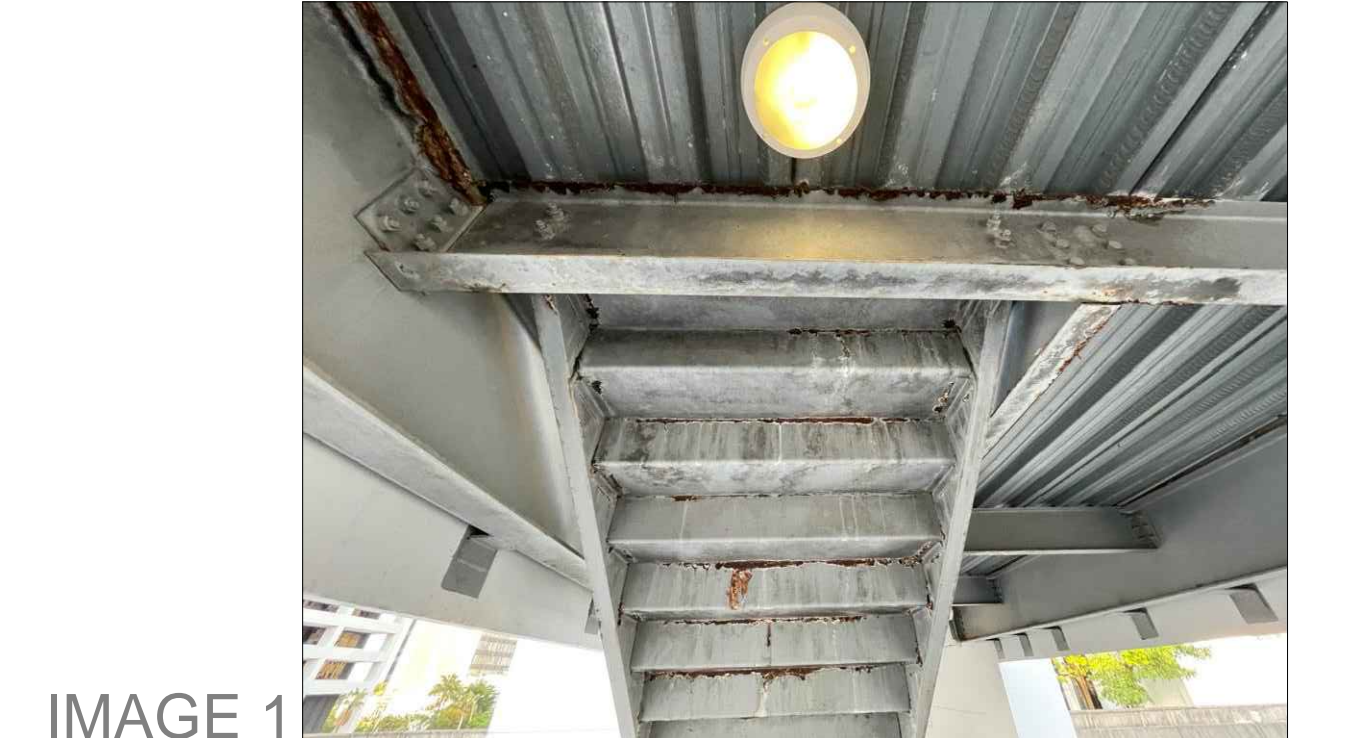
IMAGE 1 DAMAGE BEAM AND CORRODED MEMBERS
