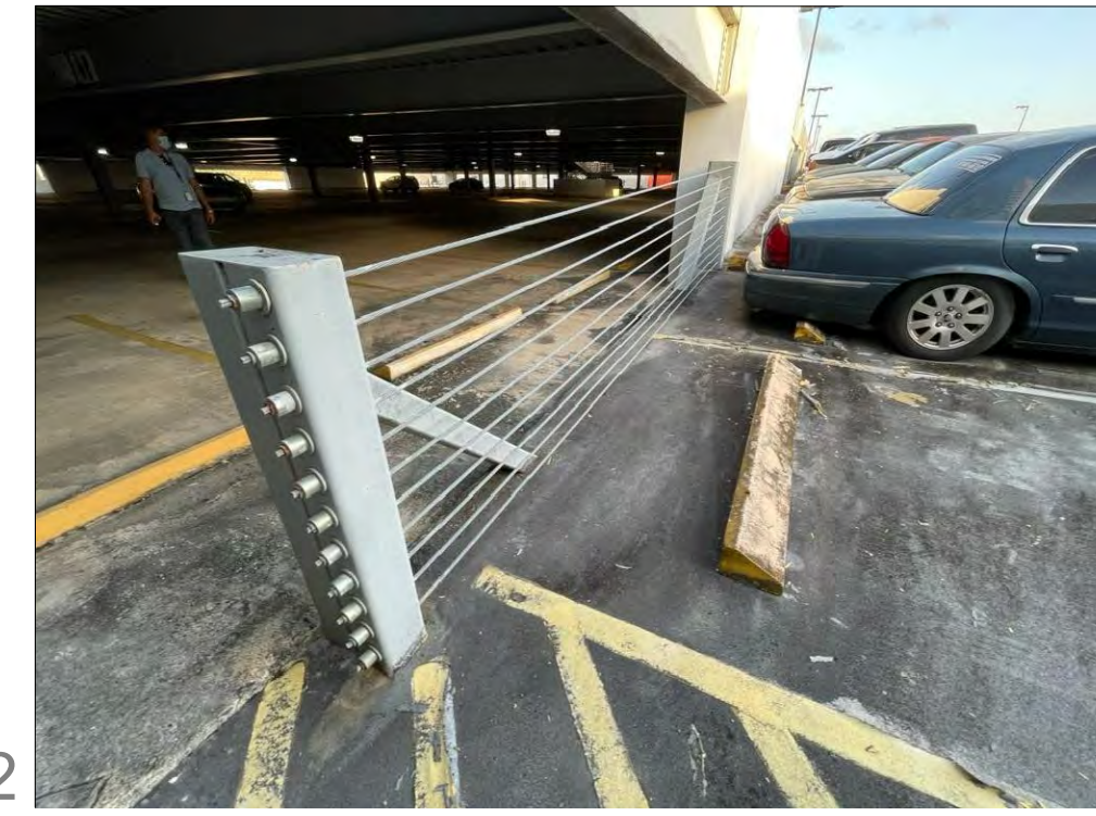
METAL POST AND CABLE BARRIER
