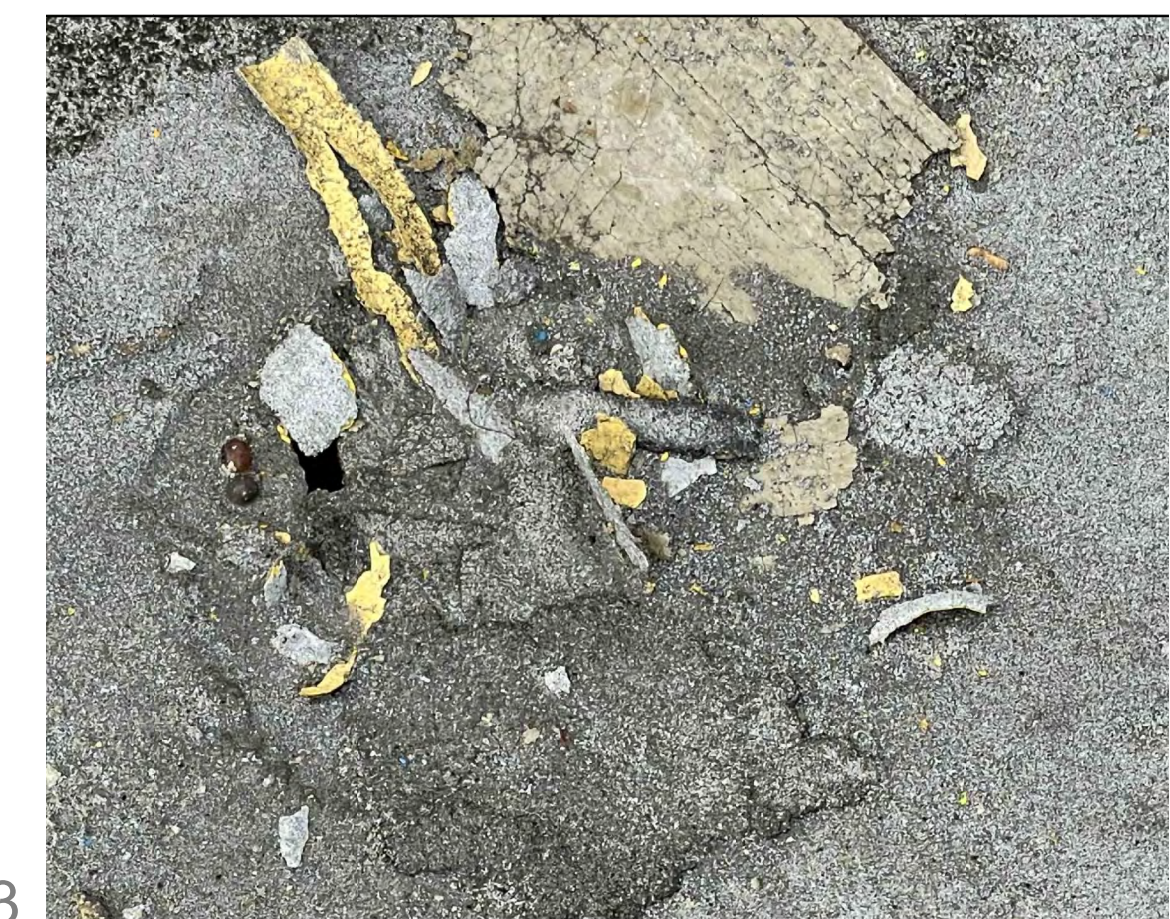
CORROSION CAUSED BY THREE EXHAUST PIPES AT EAST FACADE
